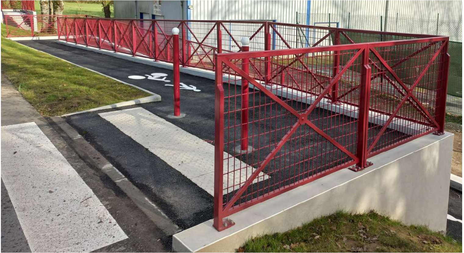
Garde-corps Croix Saint-André
